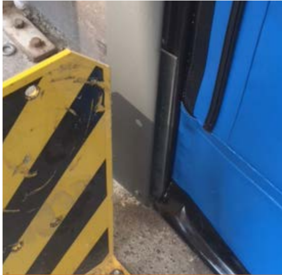
Heavy-duty zip system and FlexEdge bottom beam
