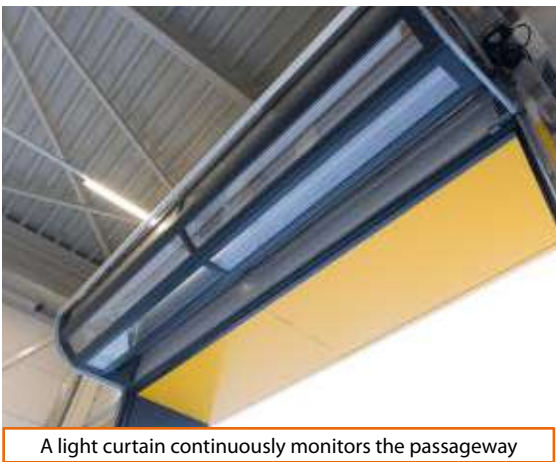
A light curtain continuously monitors the passageway
